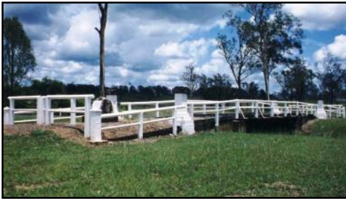
Bridge Creek War Memorial Bridge on the Brooweena-Woolooga Road
